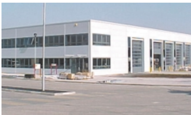
Our new test station, in North Manchester, near completion
