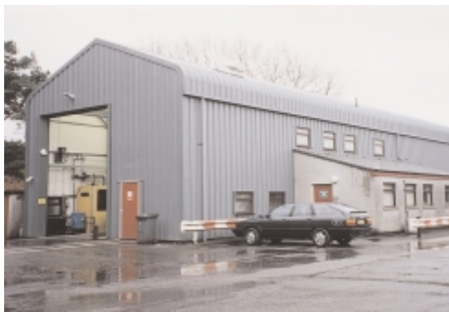
Refurbishment at our stations improves the working environment for customers and staff
