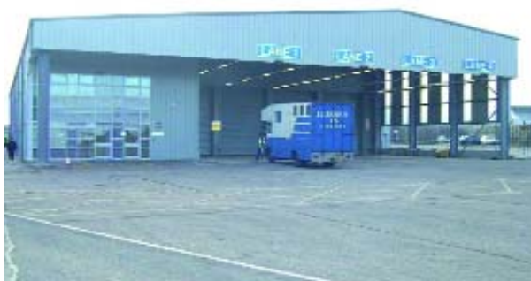
A recent refurbishment
